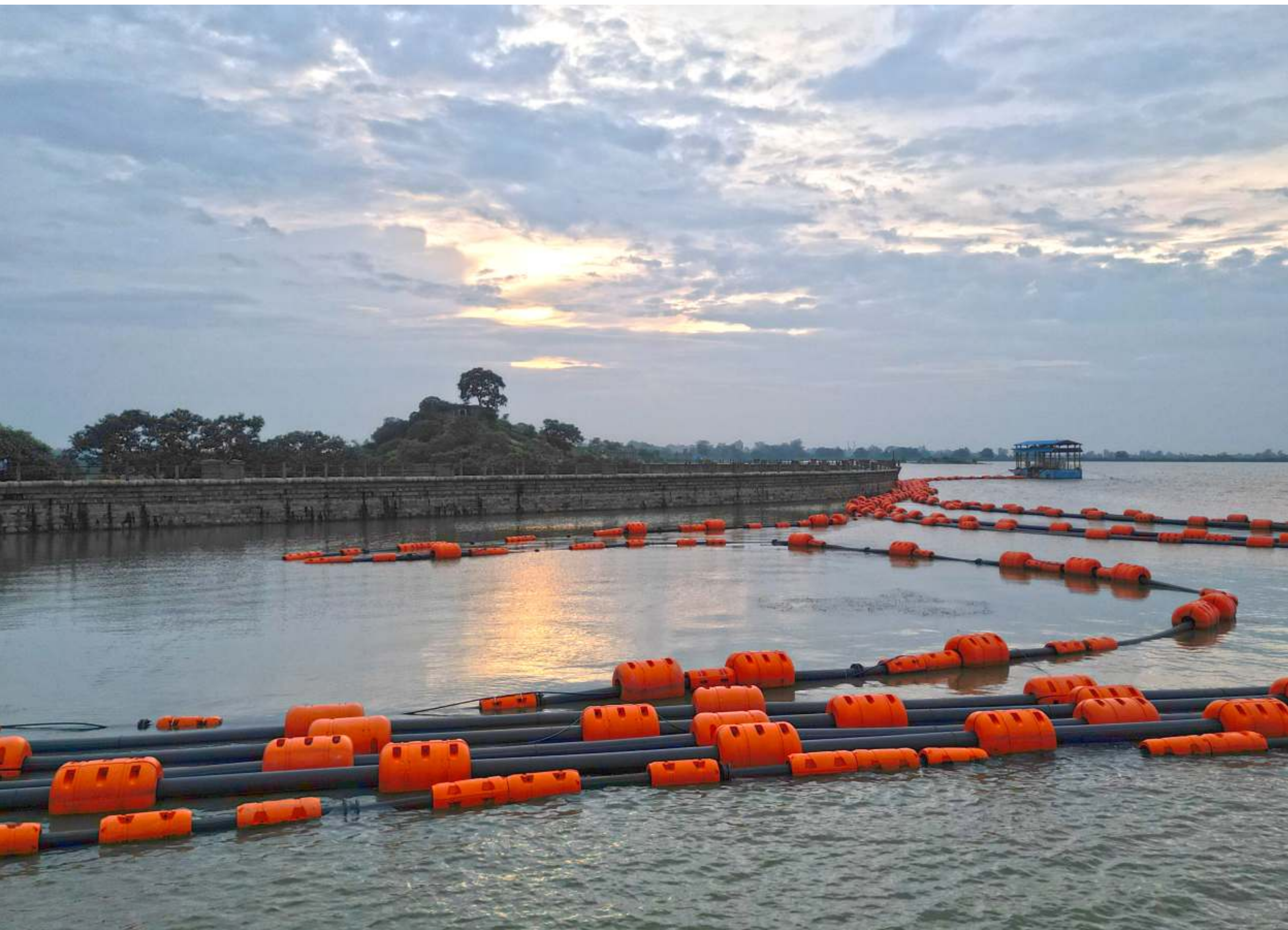
Surface Water Scheme with Floating Intake Well in Sonbhadra
