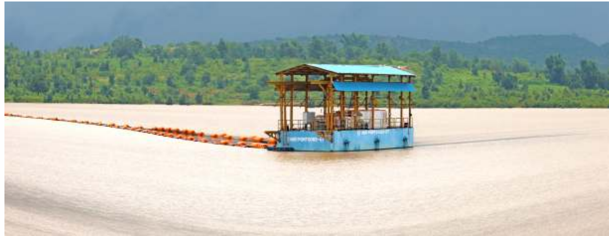
Floating Intake Well at Water Treatment Plant in Sonbhadra
